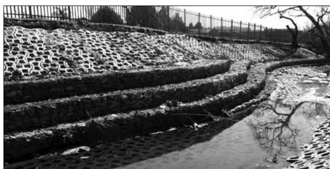
PERMEABLE HEAVY DUTY RIVER LINING
