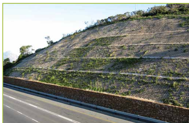
PERMEABLE SLOPE STABILISATION
