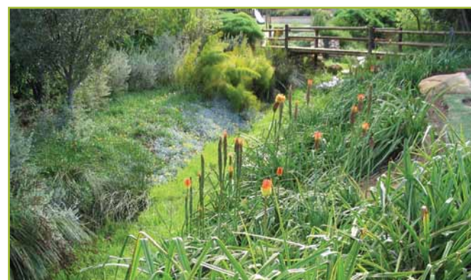
PERMEABLE STREAM LINING WITH COMPLETE PLANT COVER
