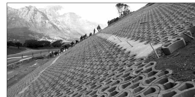
REINFORCED SLOPE STABILISATION
