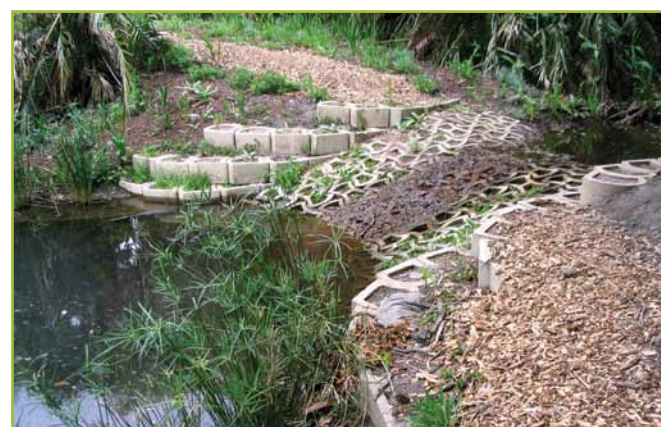
DAM SPILLWAYS AND INLETS
