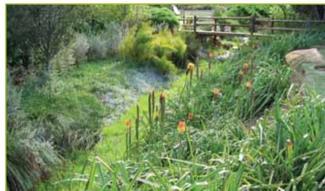
PERMEABLE STREAM LINING WITH COMPLETE PLANT COVER
