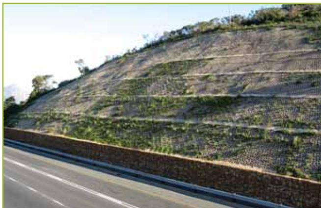
PERMEABLE SLOPE STABILISATION
