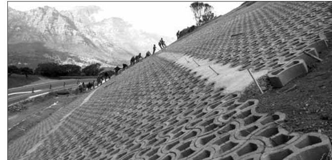
REINFORCED SLOPE STABILISATION
