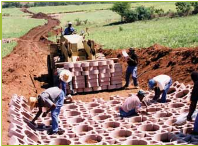
STORM WATER CONTROL IN AGRICULTURE
