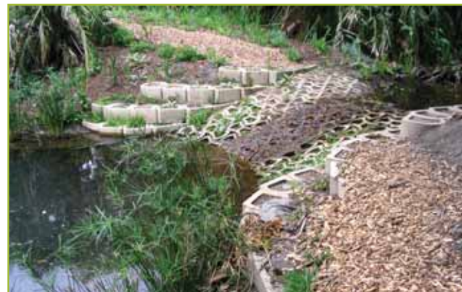
DAM SPILLWAYS AND INLETS
