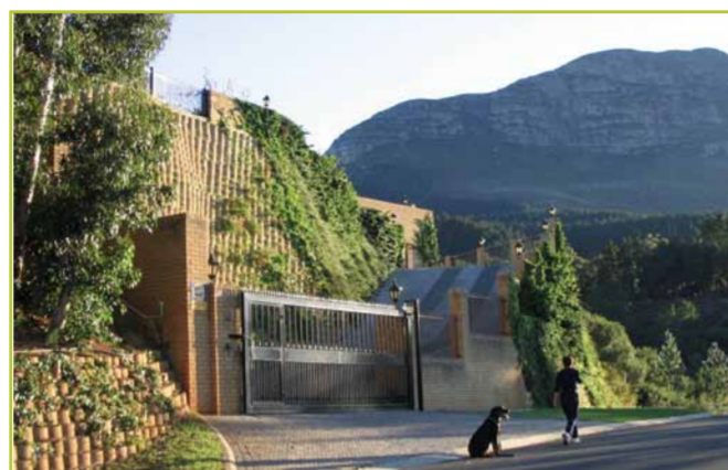
HEAVY GRAVITY WALL RETAINING, PLANT SUPPORTIVE
