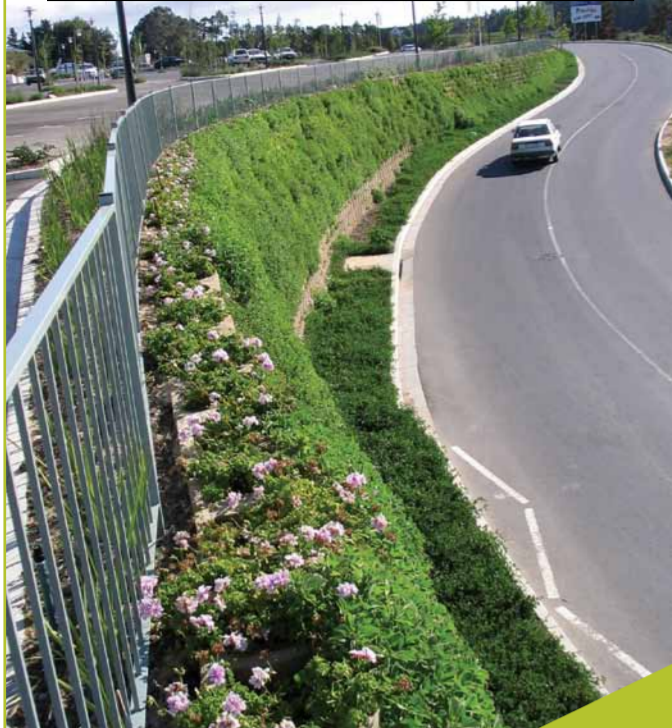
LIGHT GRAVITY RETAINING WITH STEPS, ROUND FACE FINISH
