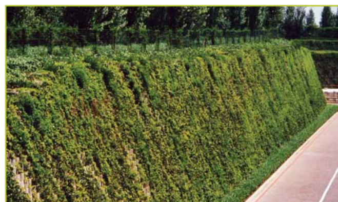
9M HIGH COMPOSITE WALL AT COMMERCIAL SITE
